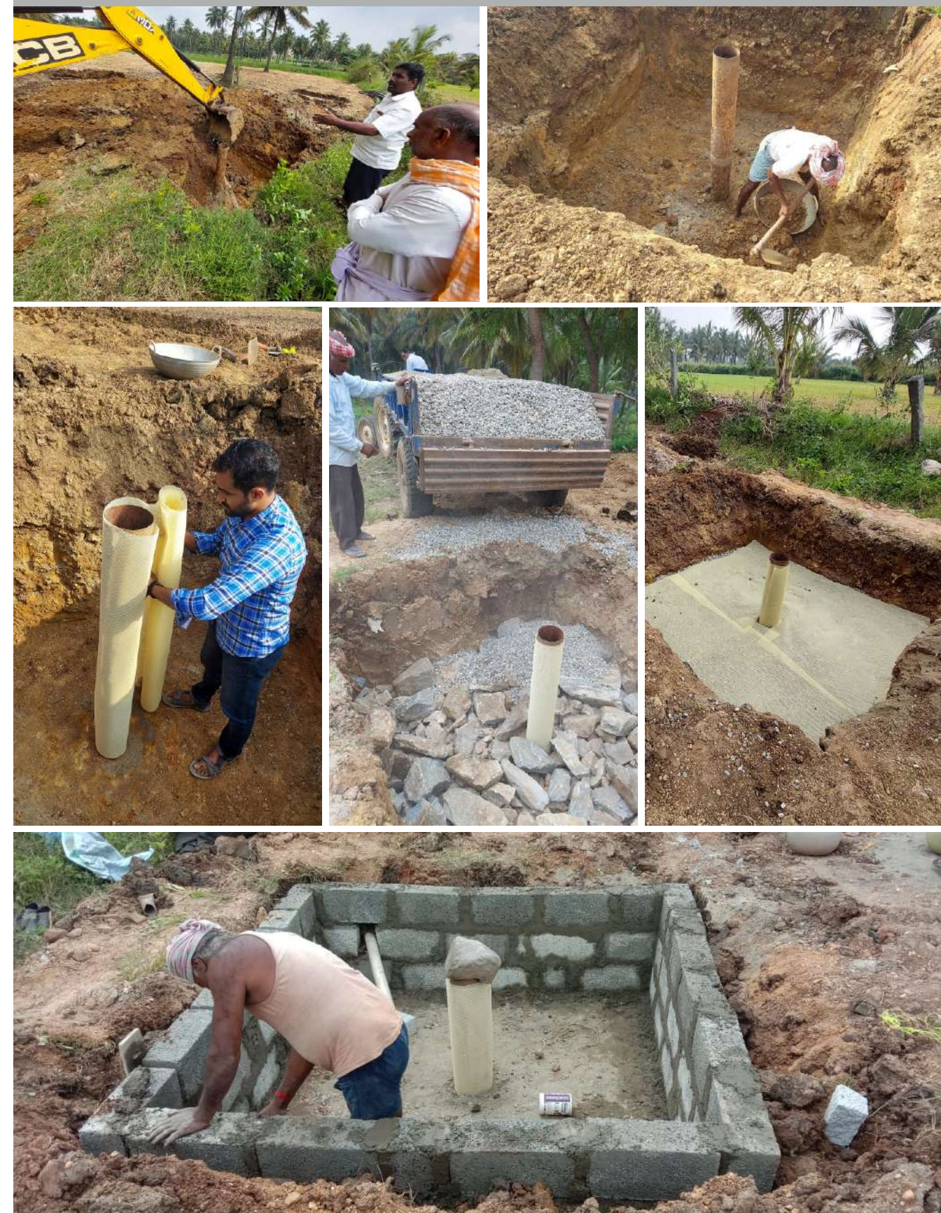
Borewell recharge pit set up village Sanenahalli
