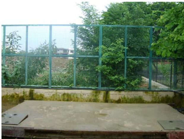
Patio 1: Completed Structure with boring
