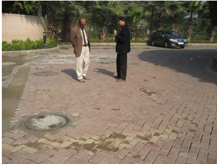
Water harvesting pits: 2 covers seen above
