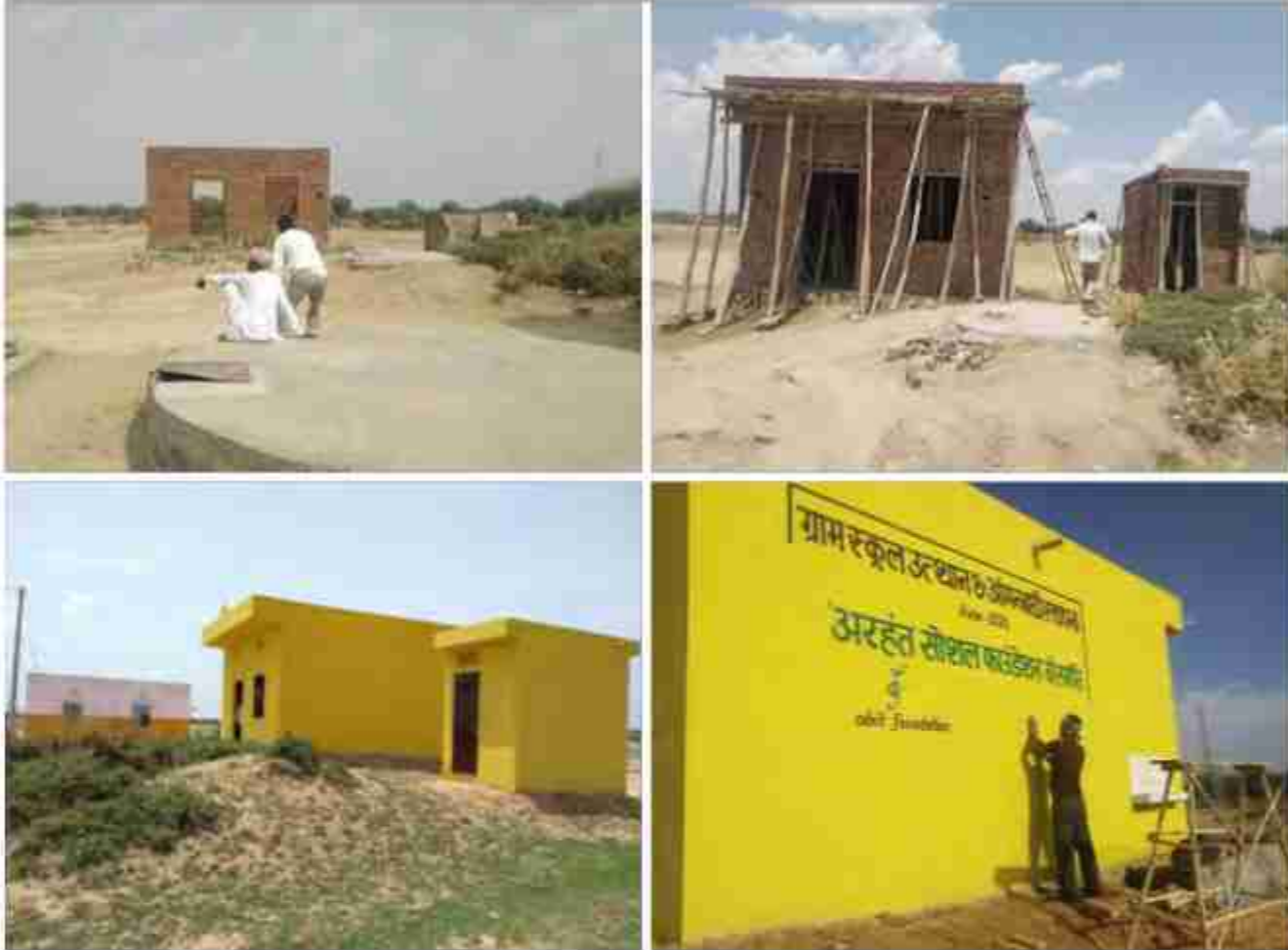
Education facility : Anganwadi construction with drinking water and toilet facility
