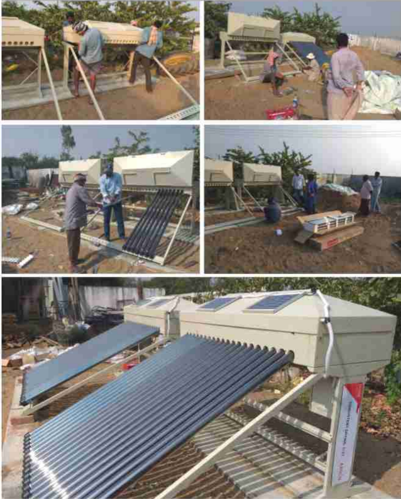
Aagun dryer installation
