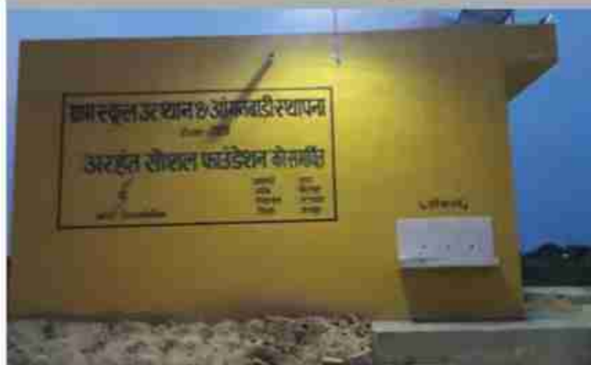
Solar electrification of Anganwadi
