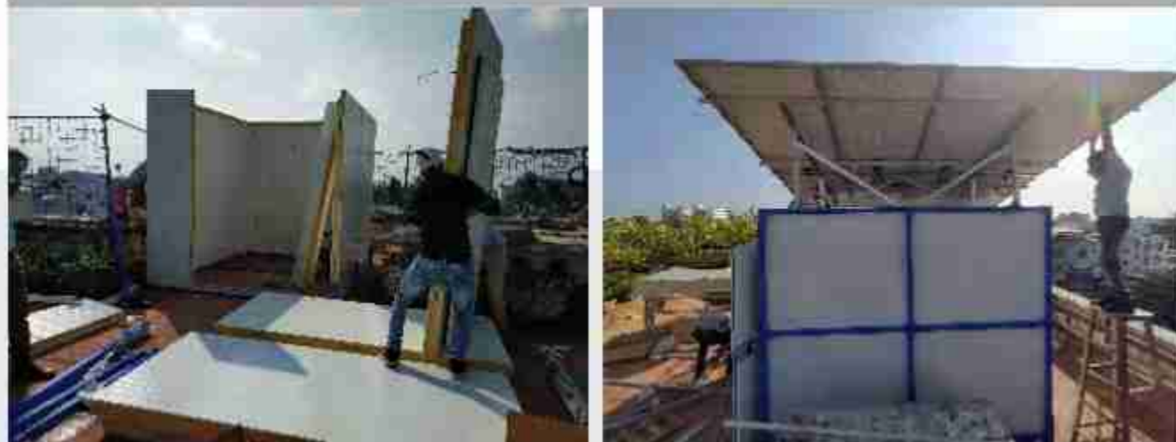
Glimpses of cold room during installation
