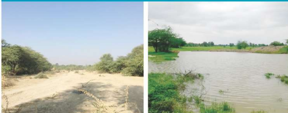
Glimpses of construction of toilets & water conservation structure in Phagi
